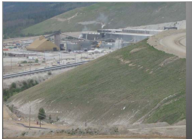
9 – Waste rock dumps are built up to specific dimensions. When reached that size and shape, they must be reclaimed (hyperlink to Mine site reclamation), re-sloped if necessary and re-vegetated.
