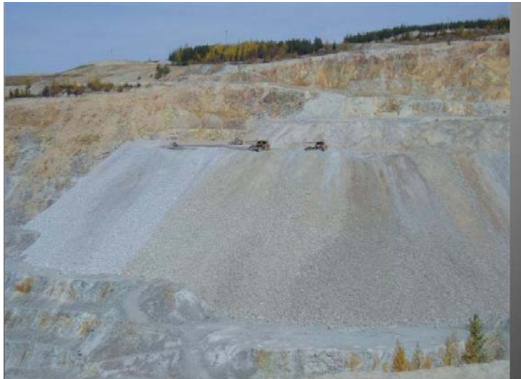
8 – The location of waste rock dumps is determined in the original mine design. They are generally located on the margins of an active pit, but later on can be situated in an inactive pit, as shown here.
