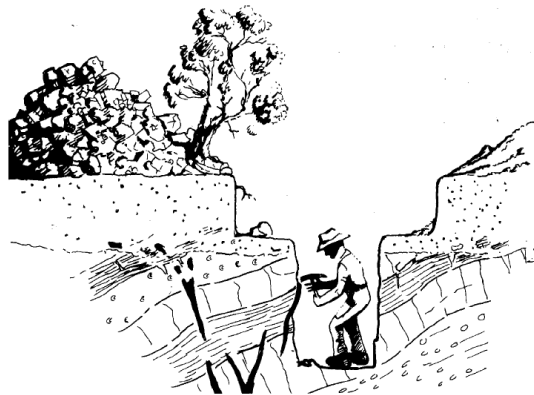
Fig. 4.1 The ideal profile of an excavator trench. Put excavated topsoil on one side of trench, bed rock spoil on the other. Stepping back the sides of the trench as shown will makes it much safer to enter
